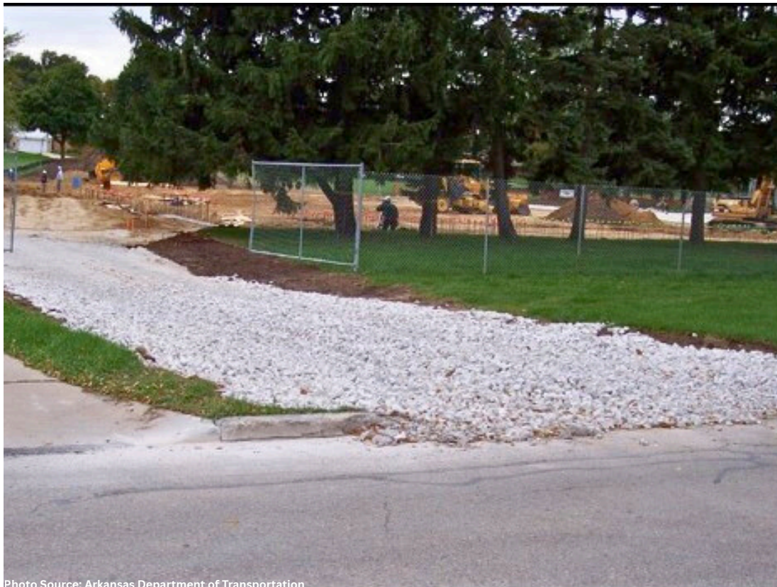
Photo Source: Arkansas Department of Transportation
