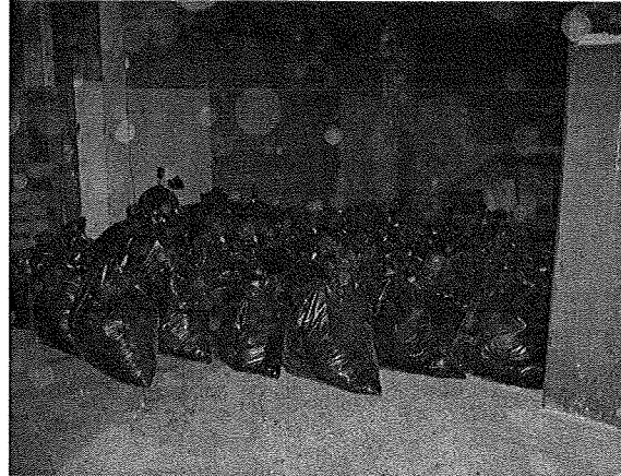
Inside warehouse —bags full of friable asbestos. The asbestos in the dumpster was bagged by workers, then moved into warehouse.
