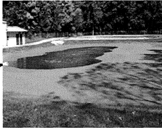
FIRST AERATED LAGOON
