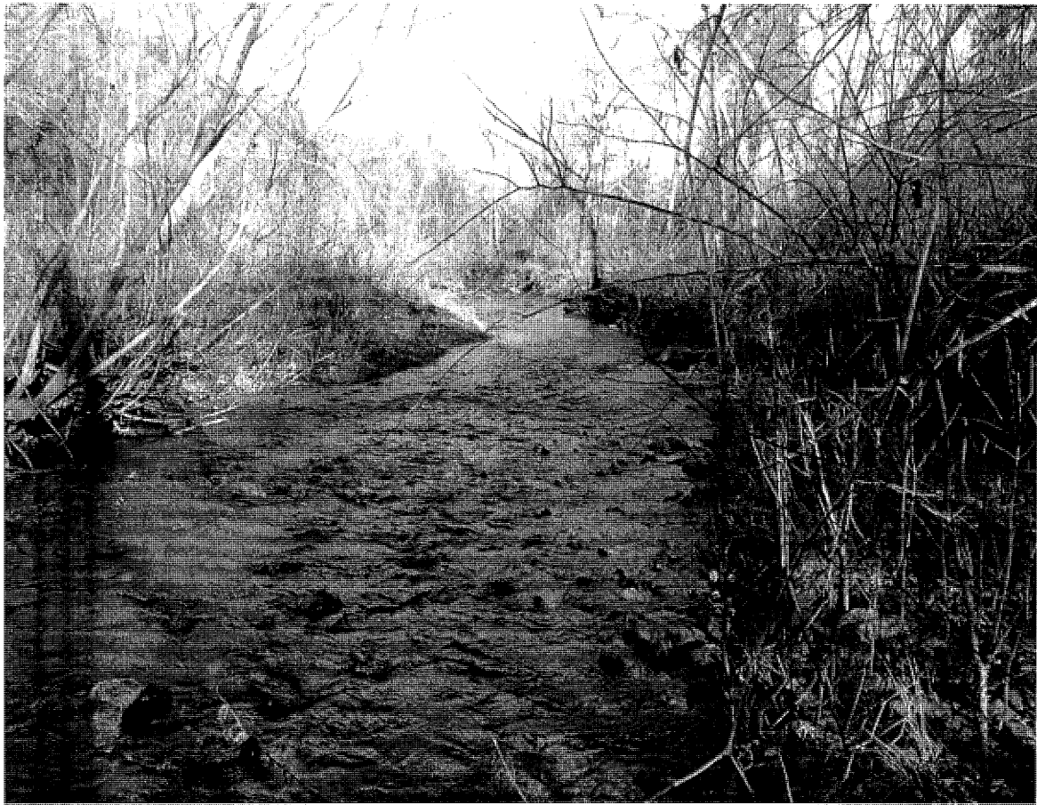
Looking downstream at Mill Creek near where 150 linear feet would be relocated
